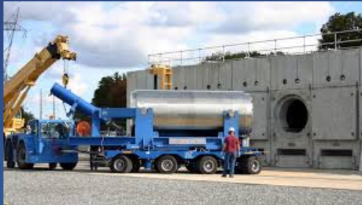
Loading spent fuel canisters into cement overpacks for long-term storage
